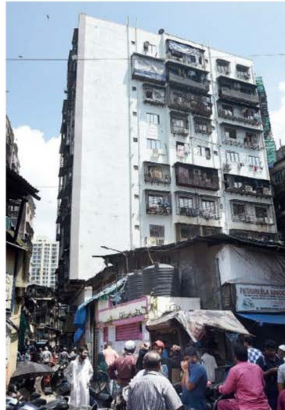
Gulistan Apartments in Pydhonie is one of the many illegal buildings
