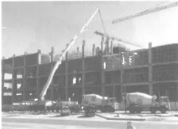
Truck Mounted Placing Boom & Pump Unit
