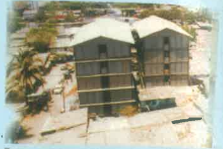
Temporary transit structure
