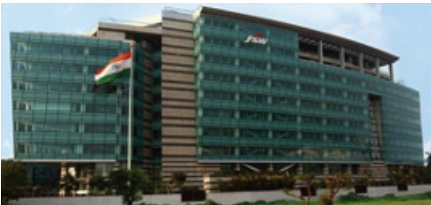
Fig.4a - JSW Headquarters, Mumbai, Office Building, Pre Engineered
