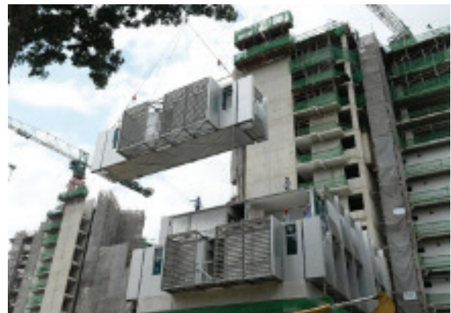
Fig.7b - Installation of PPVC Modules
