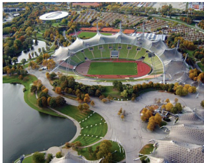
FIG 6 Munich Olympic Games Stadium - 1972
