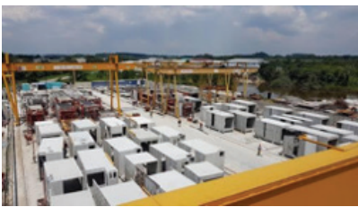
Fig.6b- Concrete PPVC Modules
