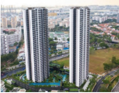
Fig.6a - Clement Canopy buildings, Singapore – Residential Building built with Concrete PPVC System
