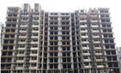
Figure 2a & 2b - Aluminum Formwork
