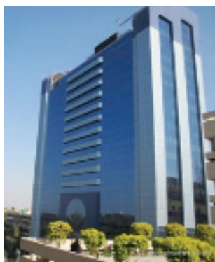
Fig.5a - IFCI in New Delhi - PEB Structure
