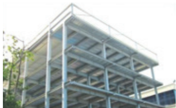
Fig.5b - Volvo Eicher Commercial Vehicles Ltd., Indore PEB Structure
